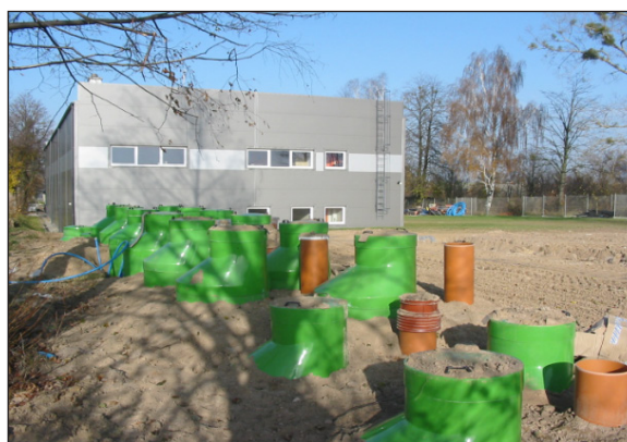
Figure 12. Research installation built in pilot plant scale
