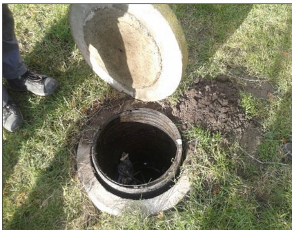
Figure 6. Condition of a manhole
